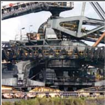
Festoon System on a Stack/Reclaimer, Australia
